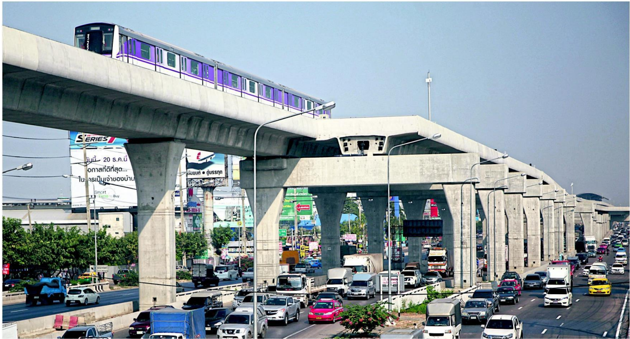
The Mass Rapid Transit Authority of Thailand (MRTA) launches a 5km test run, from the maintenance depot to Bang Yai station, of the Bang Sue-Bang Yai Purple Line. The train service will open officially on Aug 12 next year. WICHAN CHAROENKIATPAKUL
